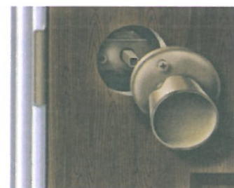
The door has a broken knob.
