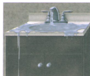
The bathroom sink is clogged.
